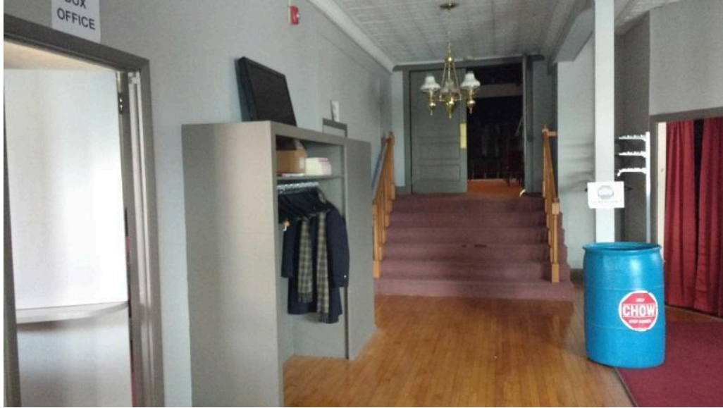
Stairs to hall, curtains on right lead to kitchen
